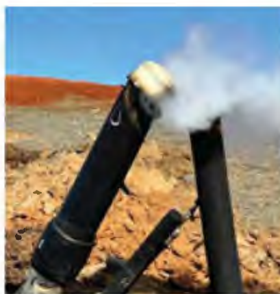
Figure 2 - Subsurface fire due to compromised infrastructure.
